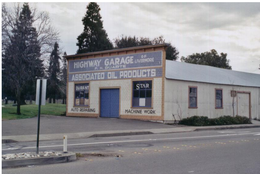
The Duarte Garage on Portola Avenue Livermore, California
