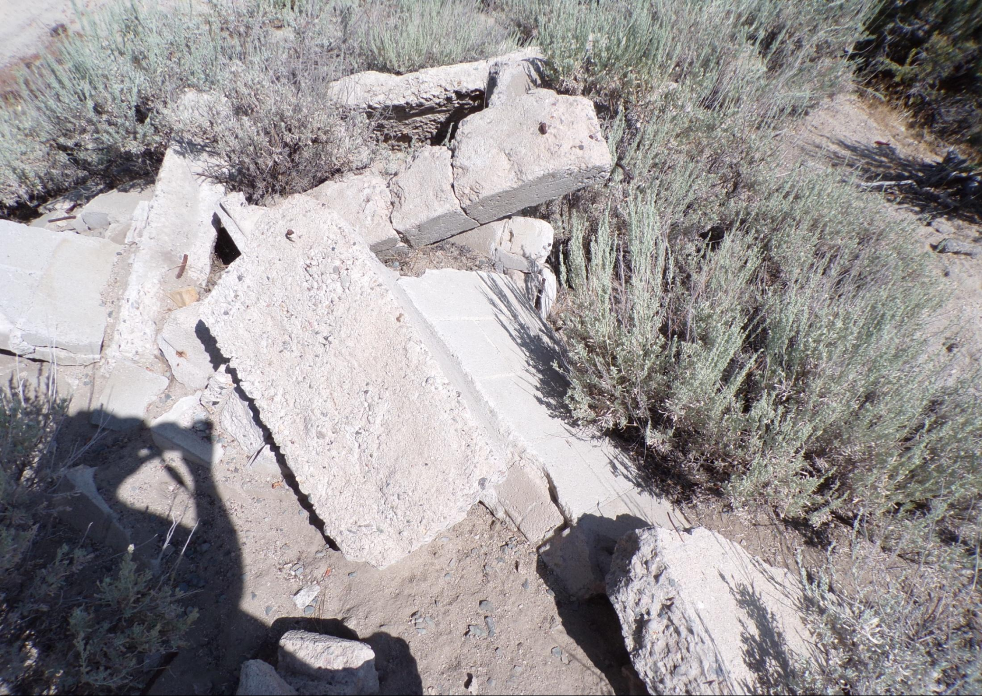
Original LH culvert-bridge, dug-up and piled as rubble along roadway.
