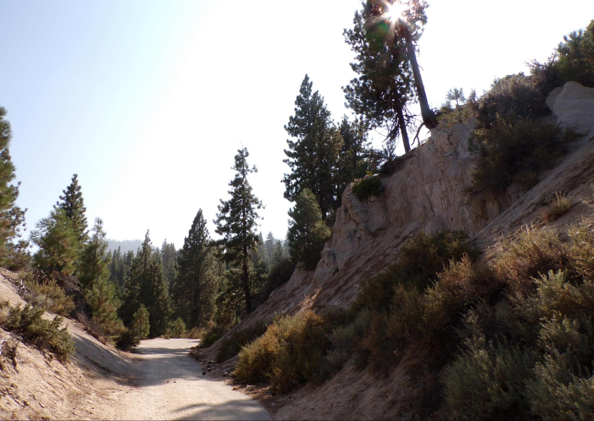
A curiously narrow section of the roadway.
