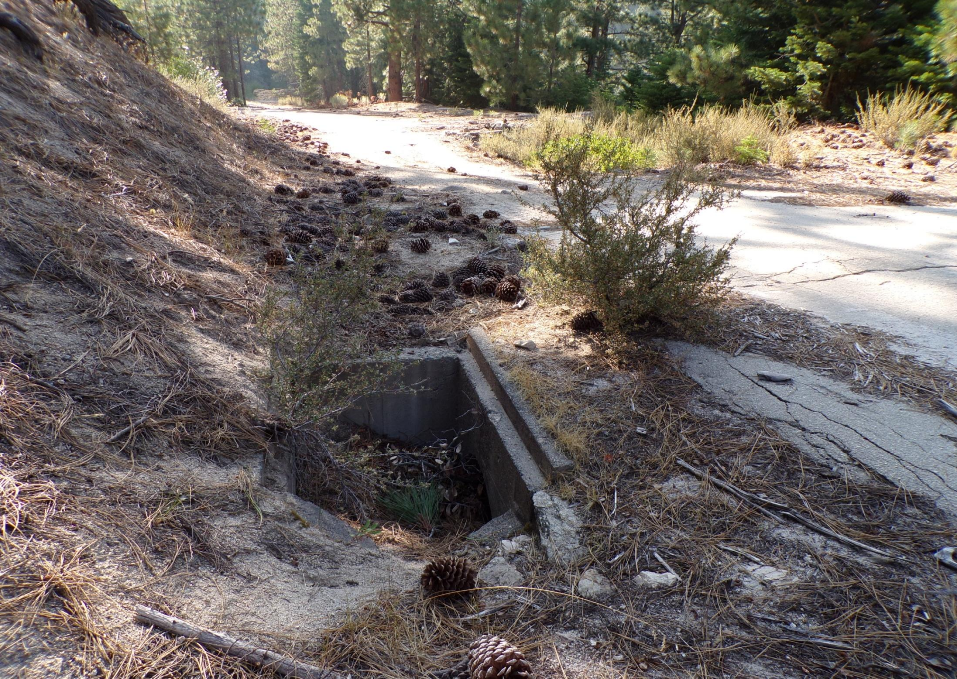
More roadway infrastructure – water-drain culvert on high-side of road.
