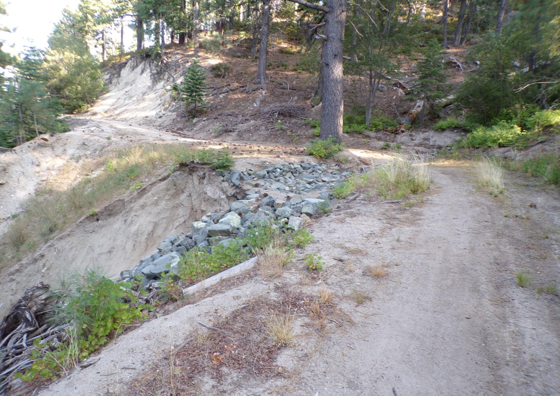
Attempts to prevent more erosion.
