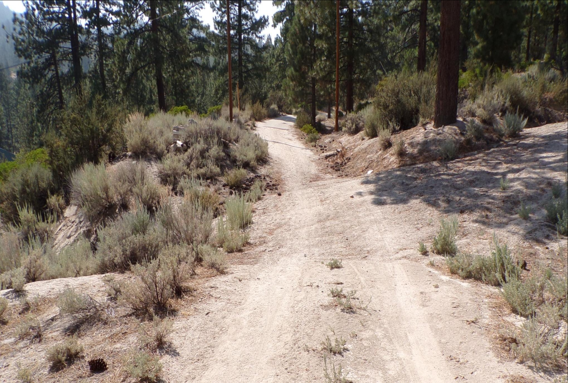
Earth covered sections – many locations. – Here due to Hwy 50 drainage gutters. Much erosion up the hill.
