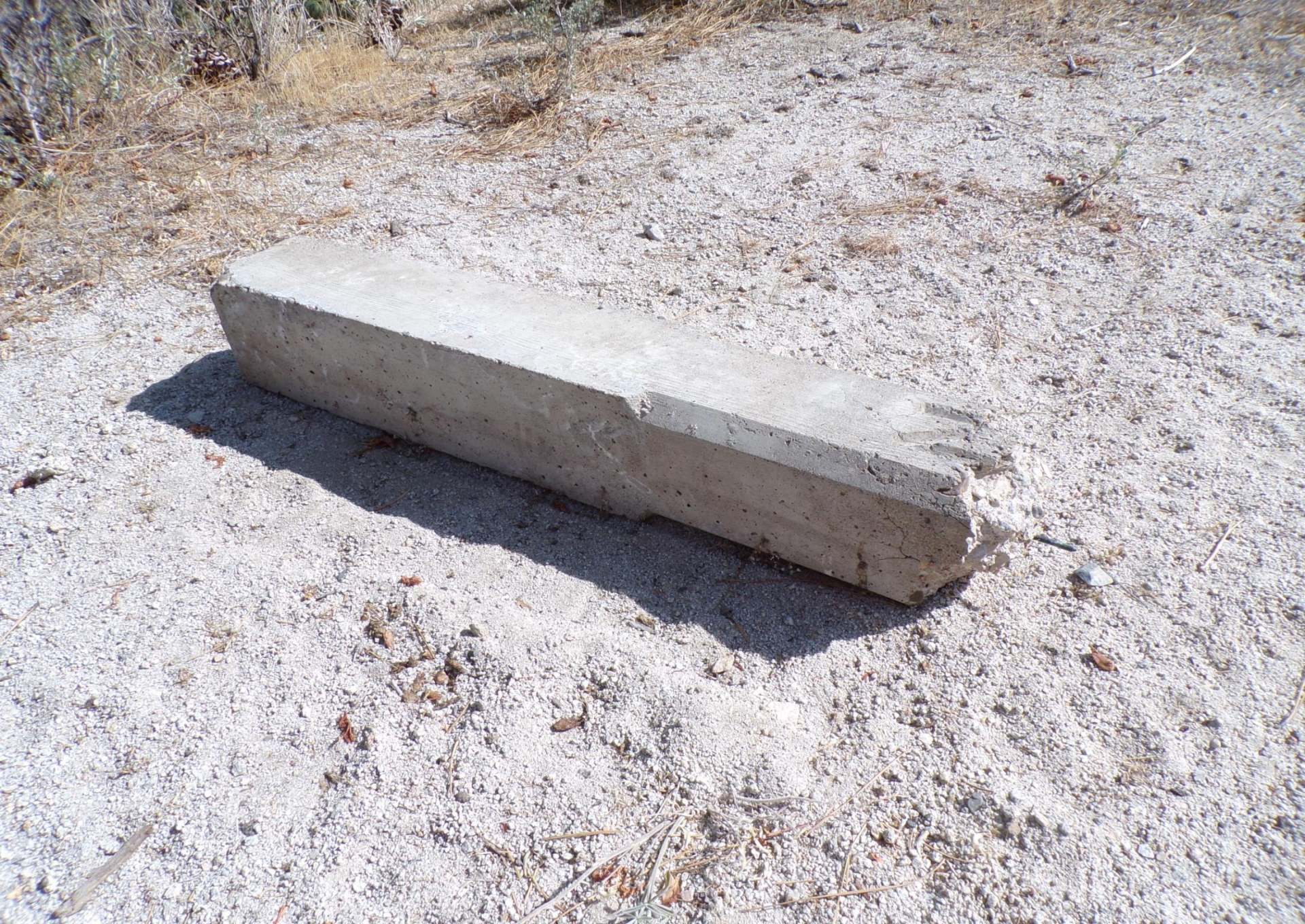
Post of a broken Nevada Road Marker
