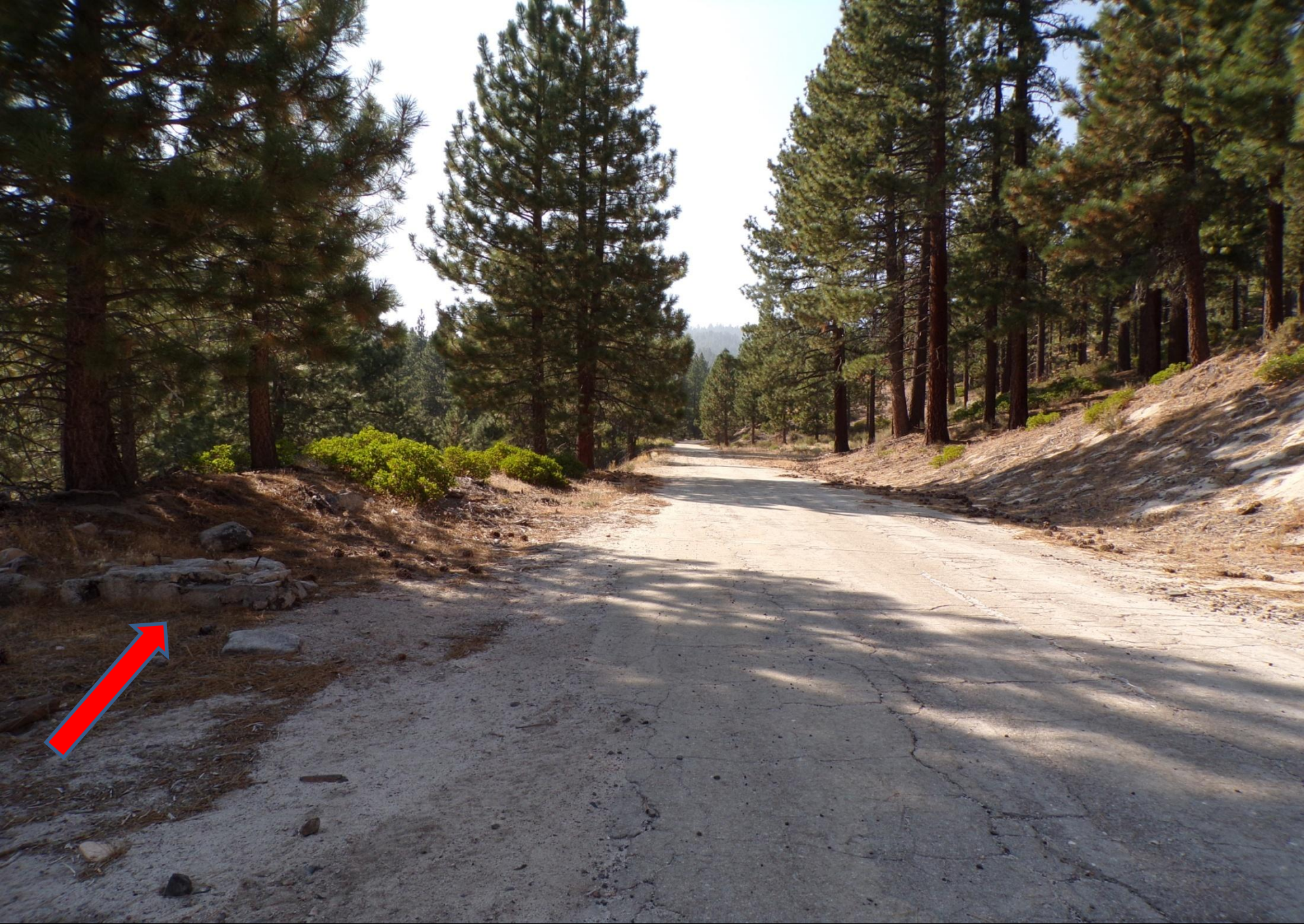
Location of Rock/concrete base.
