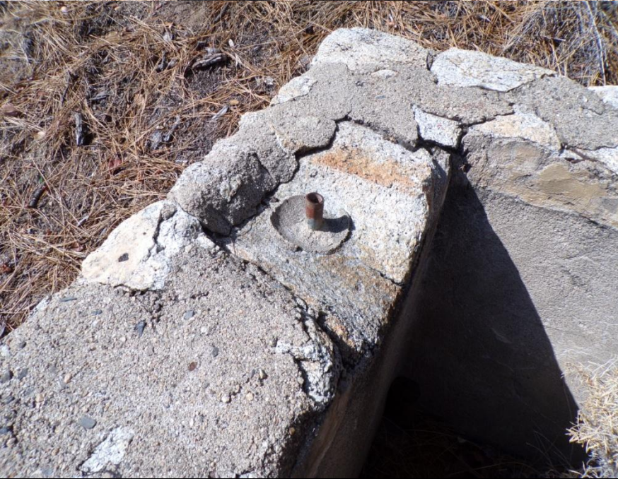
...A simple cistern to collect percolated spring water from the hill above the road.
