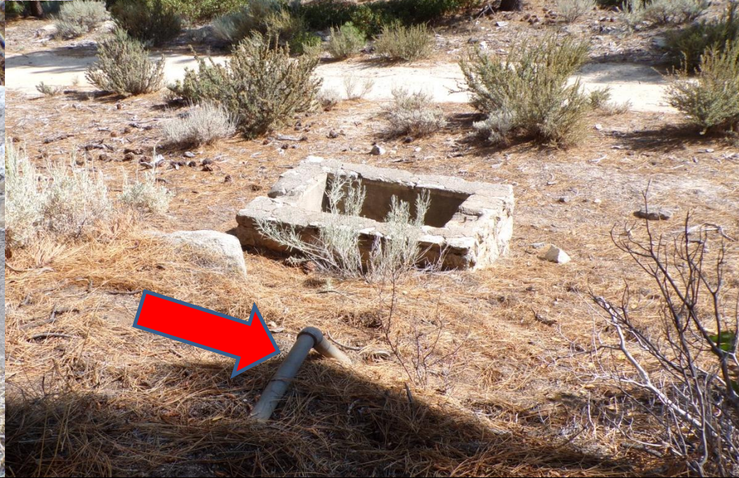
...A simple cistern to collect percolated spring water from the hill above the road.
