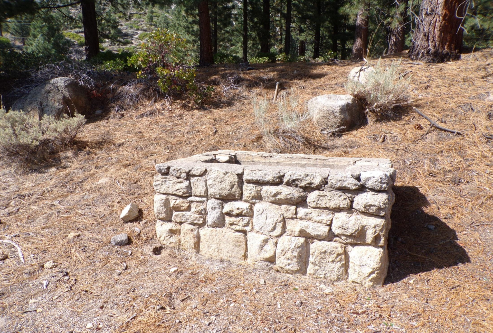
Water trough for horses and auto radiators of the day, – beautifully built and in good condition.
