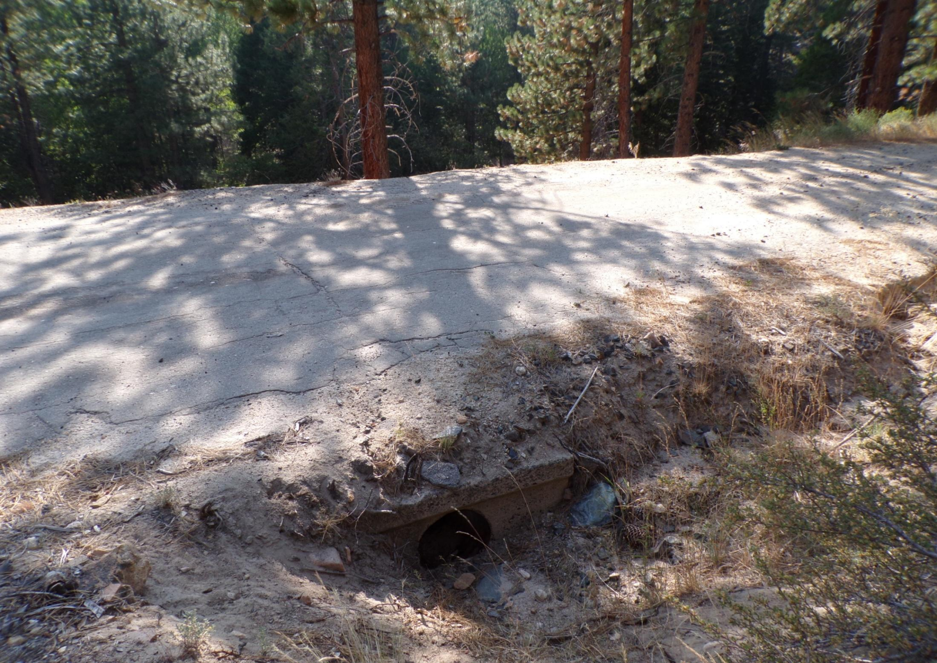
Old-road infrastructure – drainage culvert.
